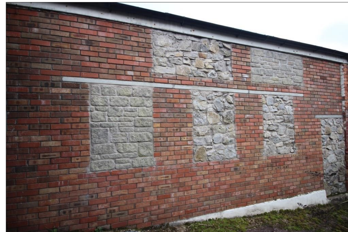
Plate 14: Northern end of western elevation of Building B rebuilt with modern brick and stone finishes
