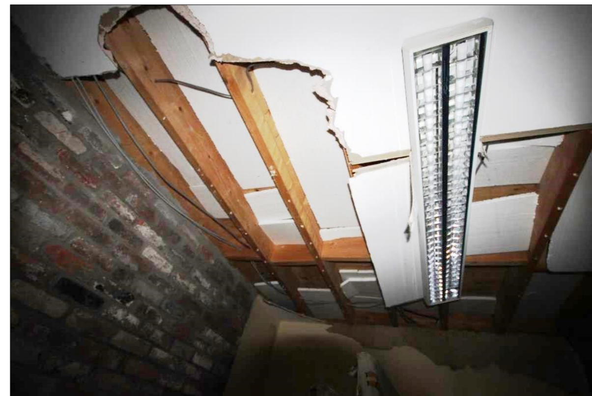
Plate 18: Modern floor joists in Building B
